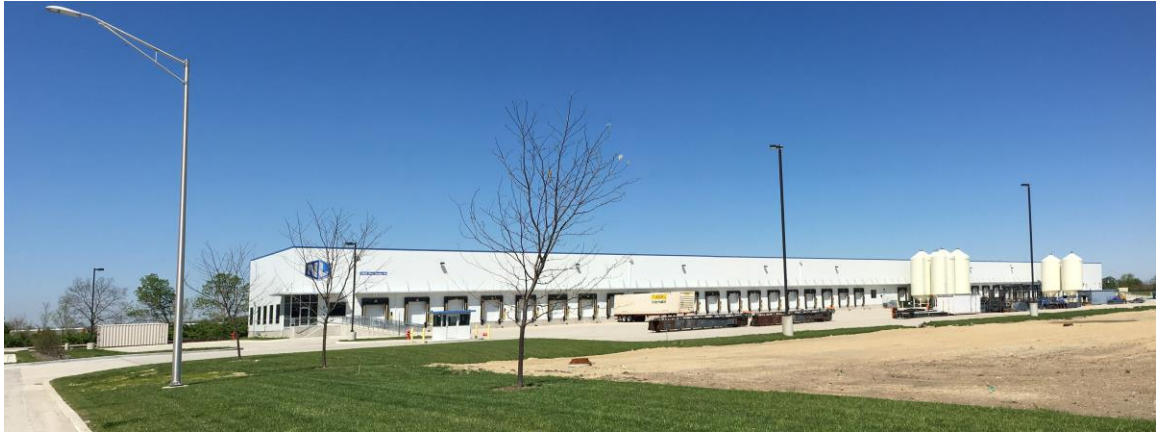
World Foods Refrigerated Warehouse
