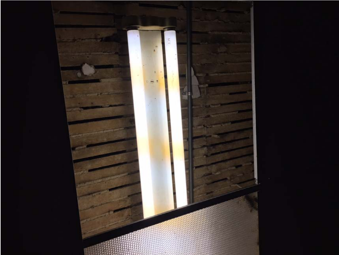
View of ceiling, second floor.
