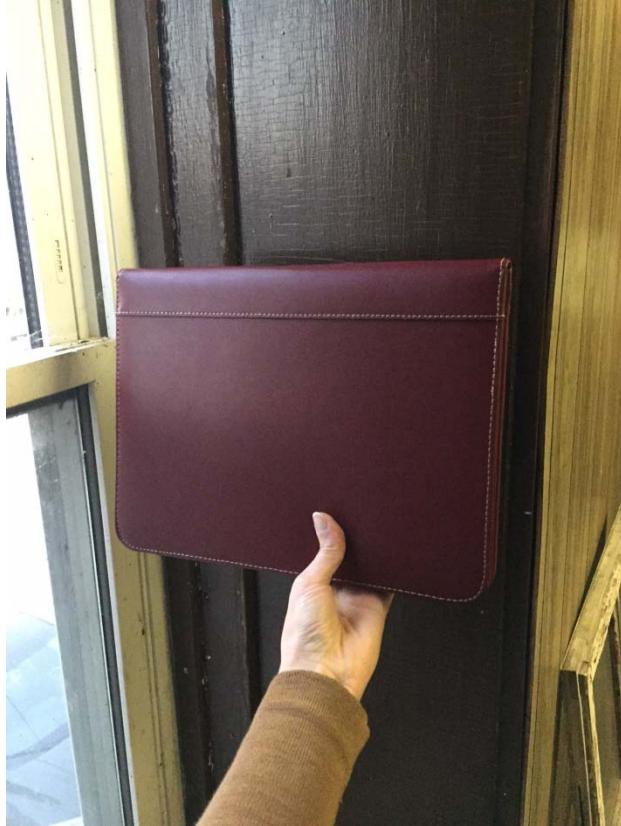
Demonstration of wall thickness, second floor.
