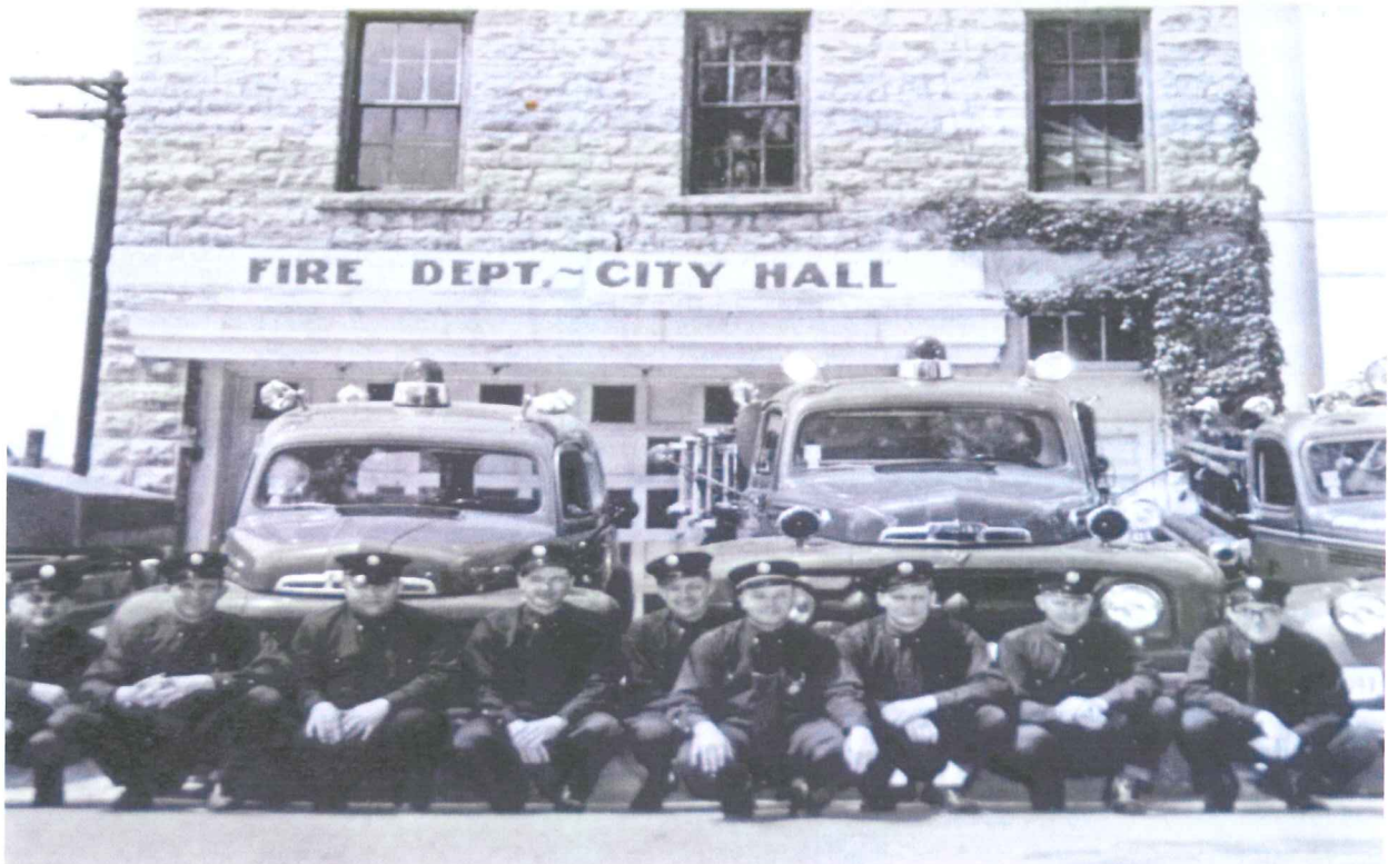
1950s-60s; note the door for fire trucks has been expanded
