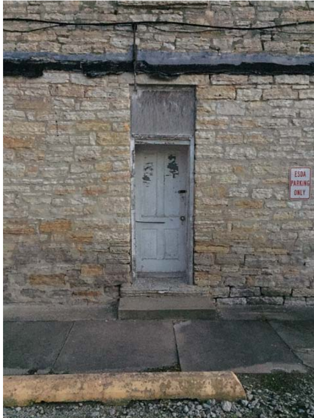
All of the exterior doors would originally have had transoms.
